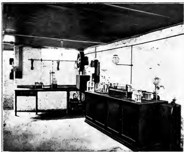
THE COMBUSTION ROOM
